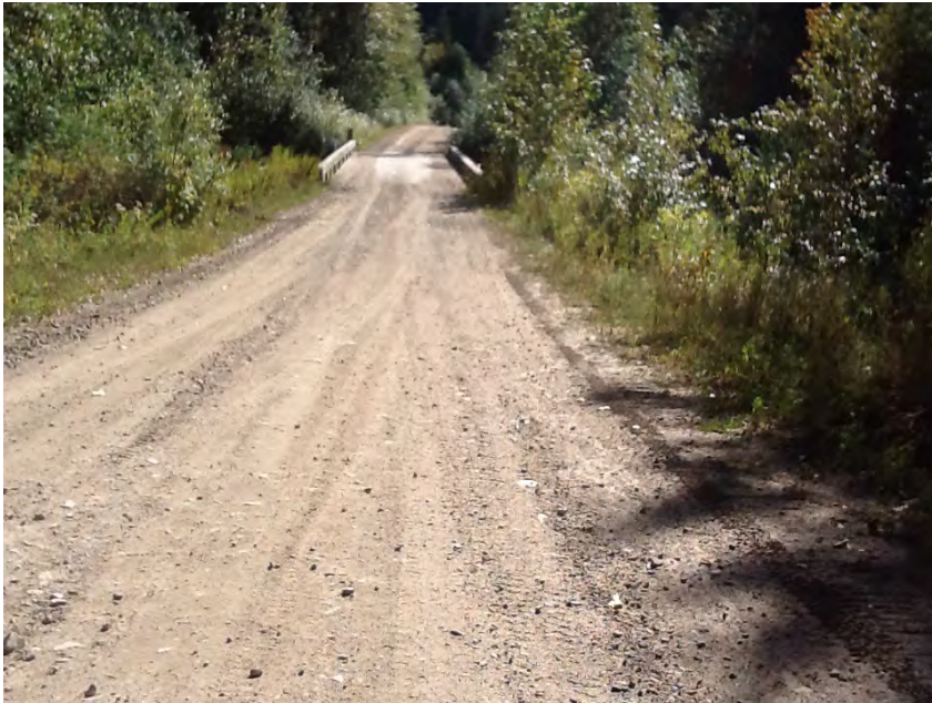
Right approach facing structure
