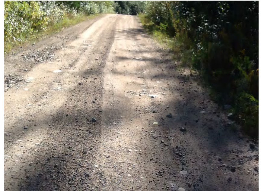
Left approach facing away from structure
