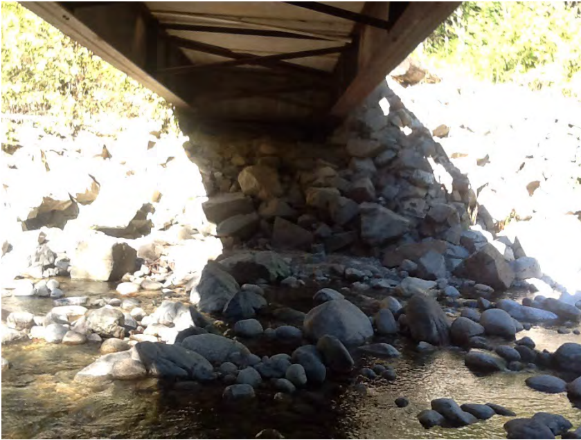
Right Bank Abutment when facing downstream
