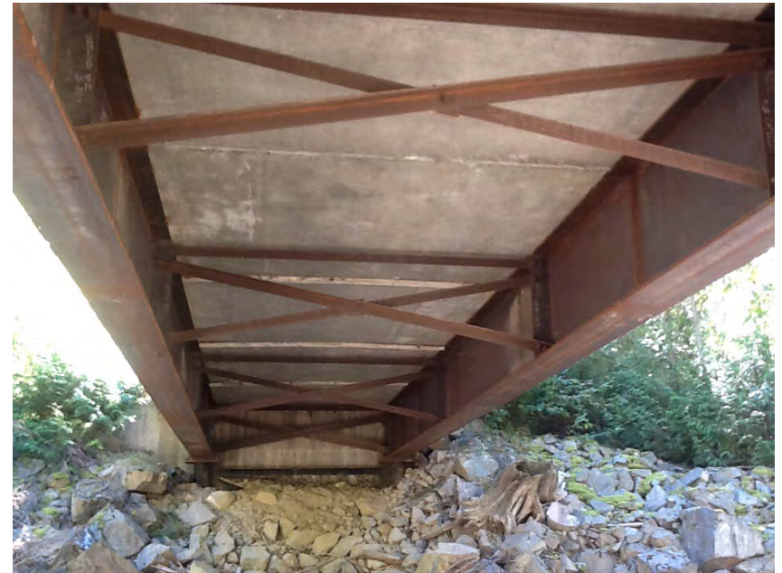
Underside of bridge
