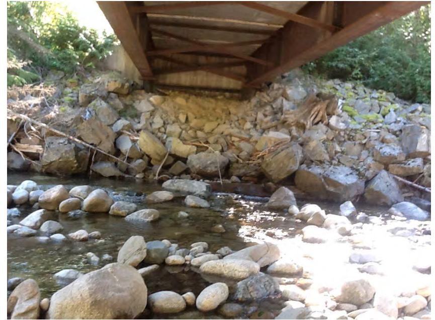
Left Bank Abutment when facing downstream
