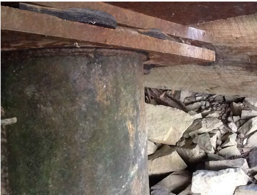
Left Bank Abutment when facing downstream
